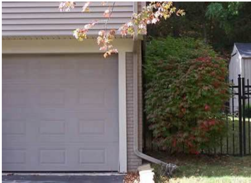
Photo 133. Downspout Disconnection, Source: USEPA
