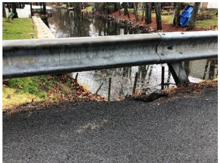
Photos 12-13. Erosion along both sides of Island Trail
