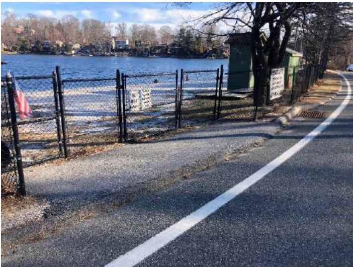
Photos 55-56. Asphalt apron and the approximate drainage area along Otterhole Road
