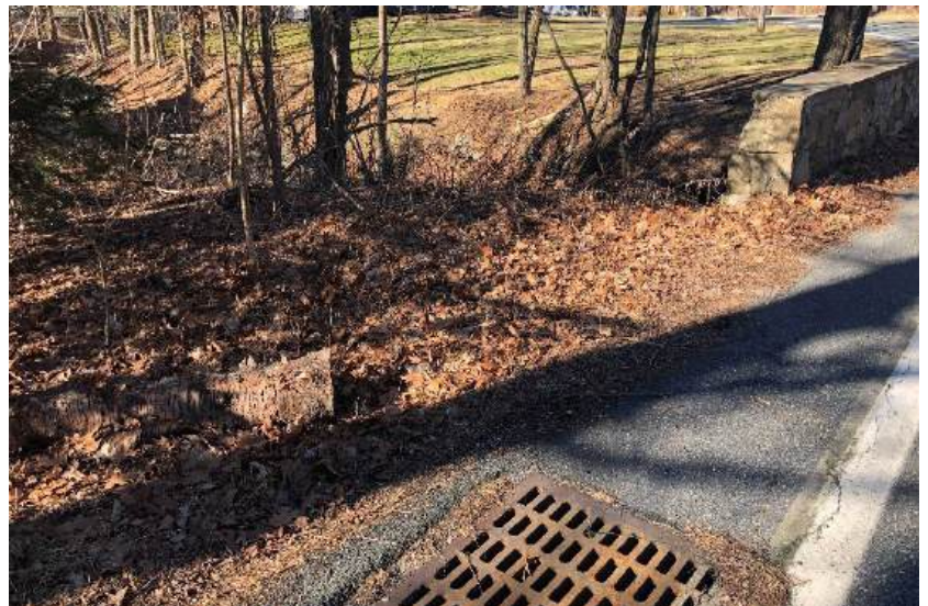
Photos 71-72. Discharge pipe from inlets up slope draining into stream (Left) Headwall and inlet on west side of Otterhole Road with debris and erosive banks and erosion at banks on residential properties
