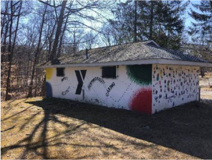
Photos 102-103. Lack of gutters on bathroom building (left) and dripline from stormwater draining off the building (right)
