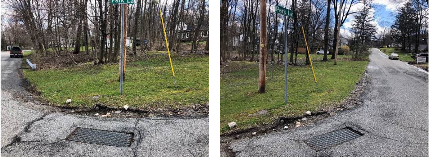
Photos 40-41. Catch basin on the corner of Pinecliff Lake Drive and Park Lane
