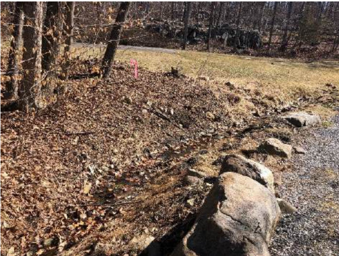
Photos 106-109. Eroded gullies to the west (top) and east (bottom) of the main inlet
