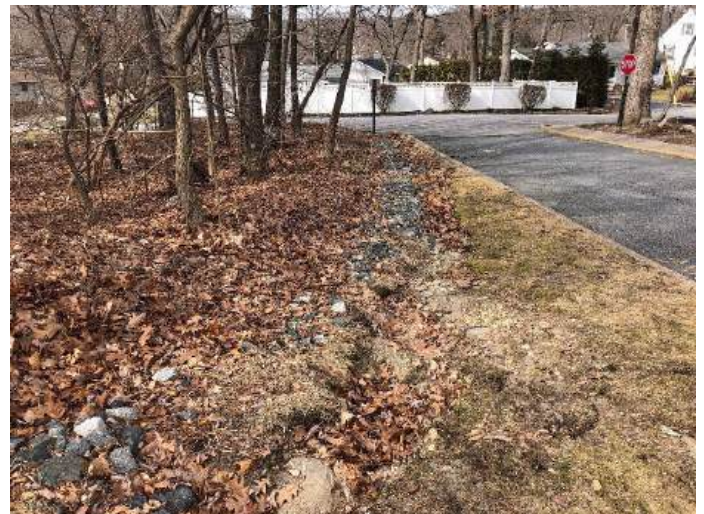
Photos 118-121. (Upper left) Looking north up long slope of parking area in front of school. (Upper right) Edge condition at head of parking stalls. (Lower left) Looking south at bottom of slope. (Lower right) Looking northwest toward Macopin Terrace- severe incising and undermining of curb from uncontrolled storm water drainage flows received from parking area.
