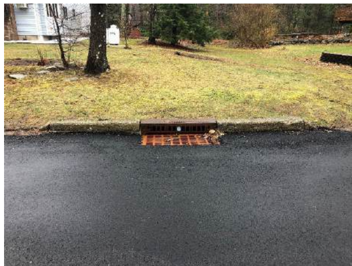
Photo 9: Catch basin on Commanche Drive
