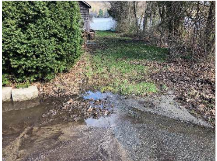
Photos 42-43. Filled in catch basin and open grass area on Pinecliff Lake Drive
