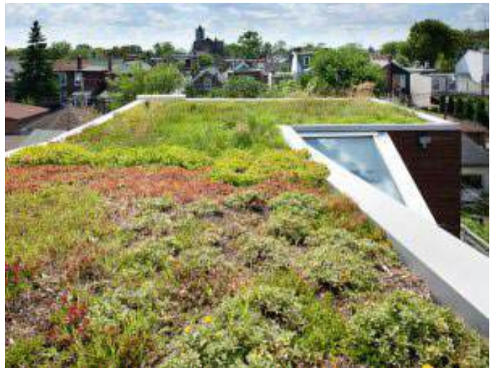
Photo 137. Green Roof, Source: New Jersey Future
