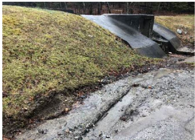
Photos 1-2. Erosion along Brookfield Road
