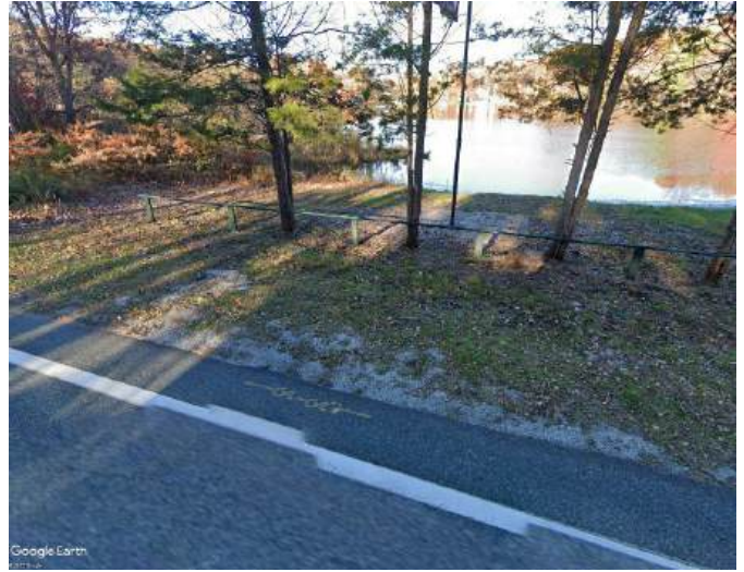
Photos 65-66. Compacted grass with pavers and flagpole (left) and visible sediment from road migrating into the lawn (right)
