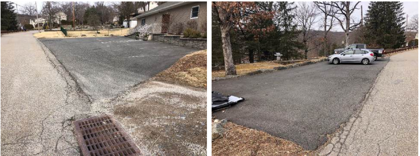
Photos 96-97. Asphalt parking lots on both sides of Forest Hills Drive
