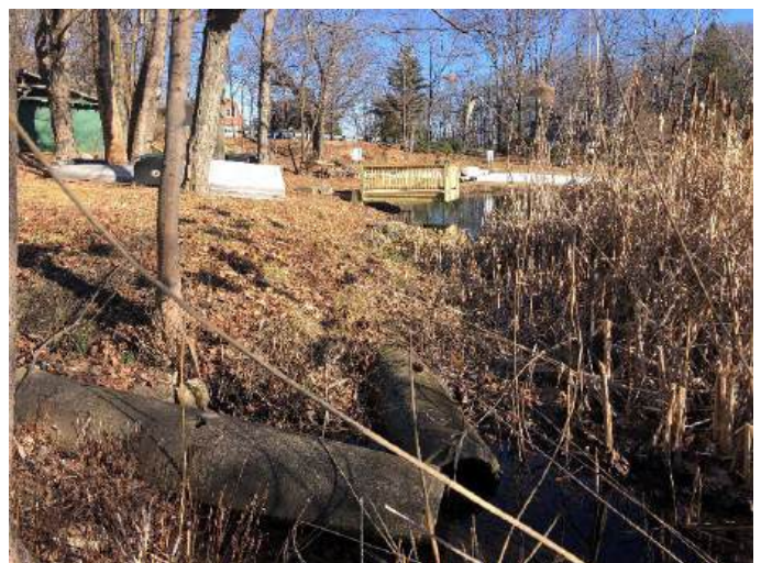
Photos 84-85. Inlet on Schofield Road that drains to lake (left) and concrete pipe ends in sediment and Phragmites stand (right)
