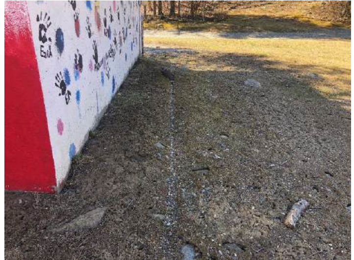
Photos 102-103. Lack of gutters on bathroom building (left) and dripline from stormwater draining off the building (right)
