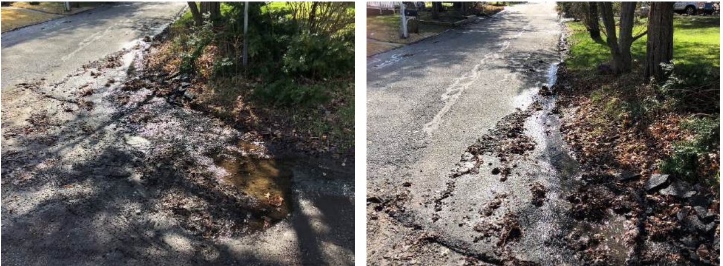
Photos 46-47. Filled in catch basin and erosion along Arcata Lane
