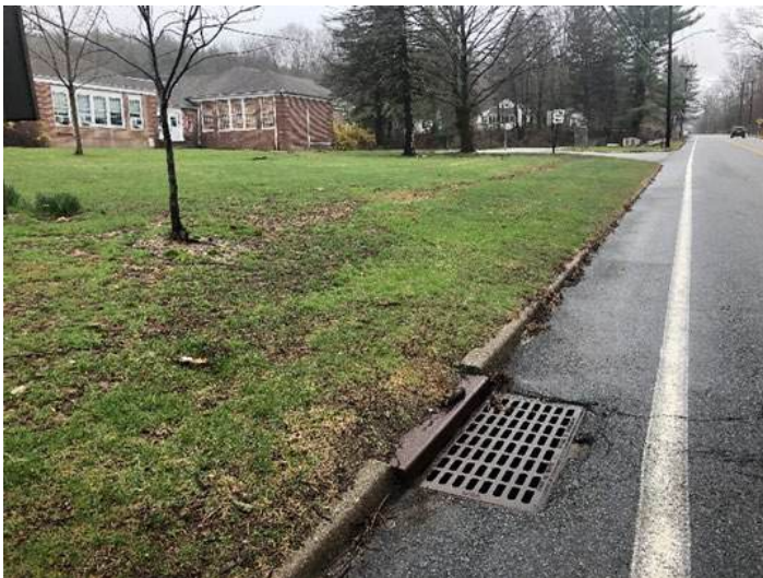
Photos 30-31. Stormwater drainage in front of the West Milford DOT building
