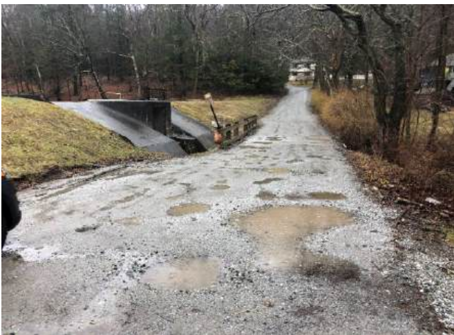
Photos 1-2. Erosion along Brookfield Road
