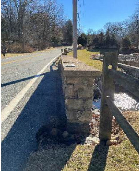
Photos 69-70. Erosion at culvert headwall and impoundment bank (left) and accumulation of sediment upstream of scour condition on west side of Otterhole Road
