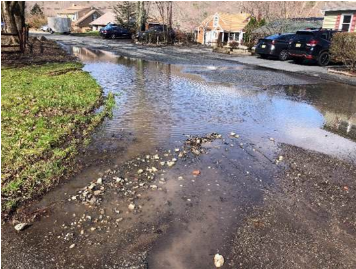
Photos 44-45. Flooding around a filled in catch basin on the corner of Sylvan Way and Pinecliff Lake Drive
