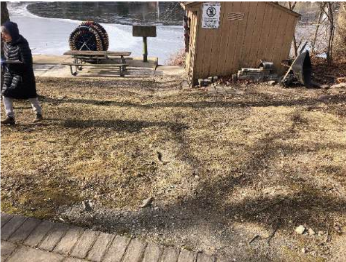
Photos 122-123. Erosion from runoff coming off pavers and running into lake and eroded area around shed (left) Impervious pavers under picnic tables and bare, compacted lawn (right)
