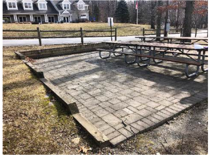
Photos 122-123. Erosion from runoff coming off pavers and running into lake and eroded area around shed (left) Impervious pavers under picnic tables and bare, compacted lawn (right)
