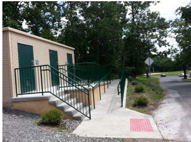
Prospect Park – Hofstra Park Bathroom construction
