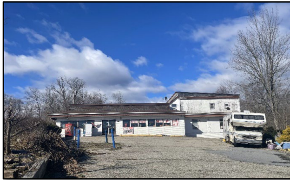
Front view of the mixed-use structure.
