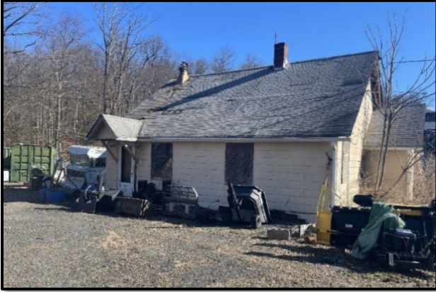
Existing, detached single-family residential dwelling
